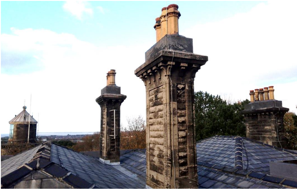
The Roof of Bidston Observatory with three chimneys.
